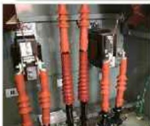
Bu-tack Mastic Putty/Tape is a self-amalgamating electrical insulation and moulding tape. This product is especially good for the use around uneven surfaces for low and medium voltage applications where connections on to busbars and bushings need to be insulated and to create a smooth profile on these connections.
