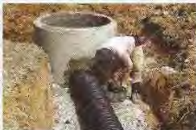
Grouting WEIDA DWCP to a concrete manhole
