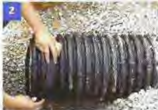
2 Insert rubber ring onto second valley of the pipe
