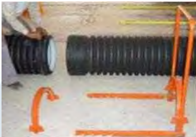
Bring pipe ends close and mount jointing device
