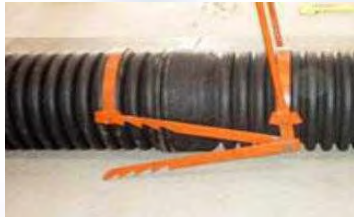
Pushing ends to fix the pipes
