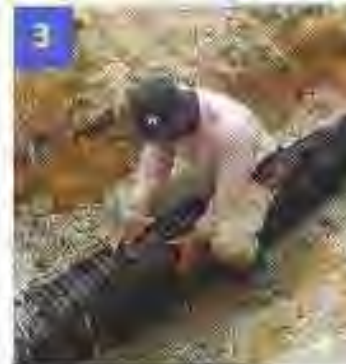
3 Push the pipe into integral bell end
