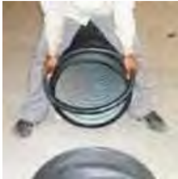
Put elastomeric ring on first corrugation
