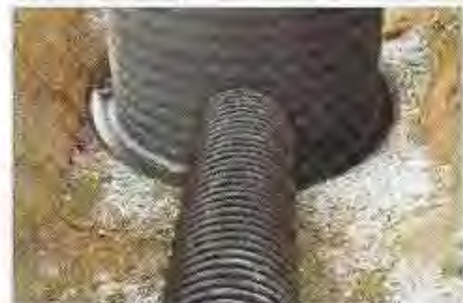
Connection of Weida DWCP to Floline 3-W manhole
