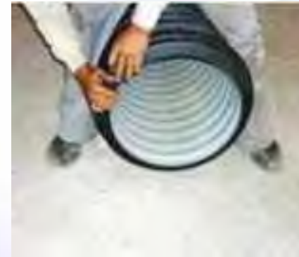
Ensuring ring is placed properly
